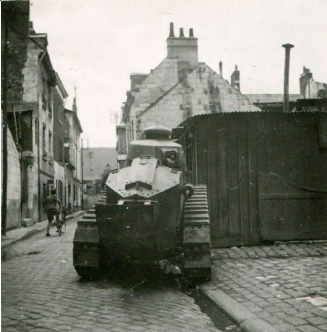
Abandoned FT-17 somewhere in France 1940
